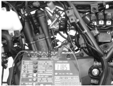
AISV working voltage measurement
