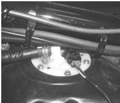
Fuel pressure measurement demolition - fuel pump
